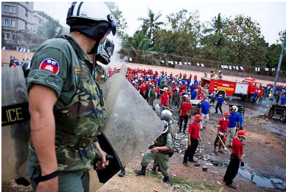
Protected by police, a horde of demolition workers (in red & blue) pour into the village. (© Peter Harris - Fotojournalism.net)
