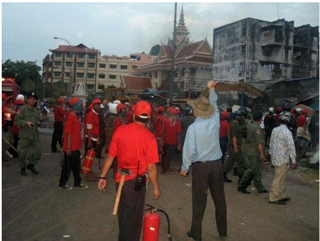
A 7NG company worker (in hat) signals for hundreds of demolition workers with machinery and tools to move in to start demolishing villagers' homes.
