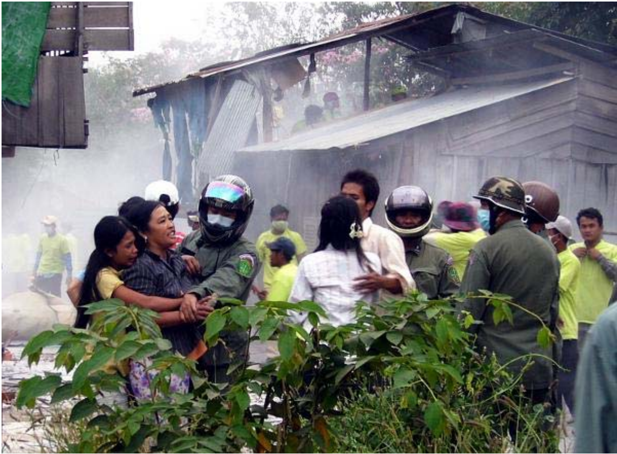
Police move residents away as demolition workers (in green) continue their work.
